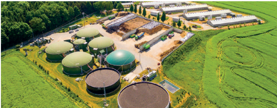
Figure 4. Biomass power plant (Energy Power Plant, 2022).
