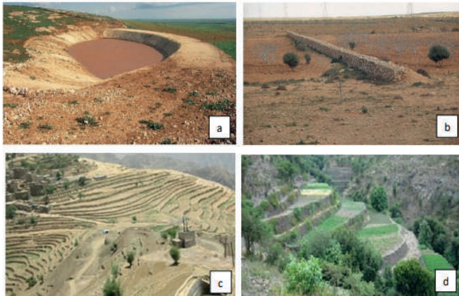
Figure 3. Micro Water Collection Systems (Ekinci, 2015); a) ridges made at the ICARDA research farm in Syria), b) Semi-circular embankments lined up in stages on the land, c) Loss system, d) A landscaped land with Negarim
