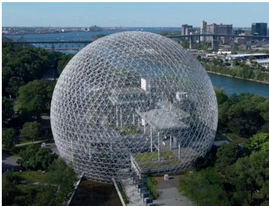
Figure 2. The geodesic dome built in 1967 by R. B. Fuller at the Montreal Fair.
