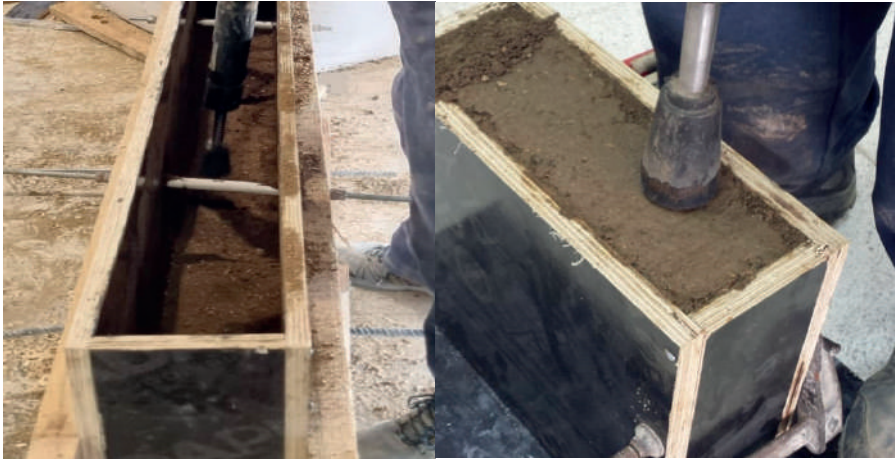
Fig. 3 Construction stage of rammed earth with modern pneumatic rammer.
