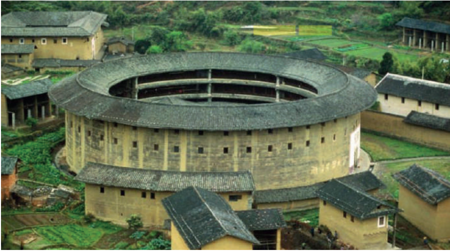
Fig. 1 Rammed Earth has been used for two thousand years in China (Easton, 2007).
