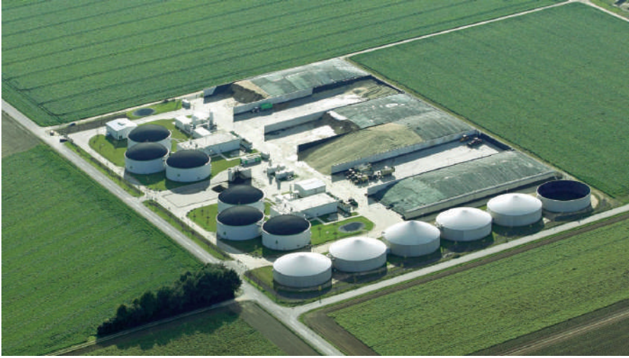
Figure 5. A biomass power plant (Piyasaanketi, 2015)
