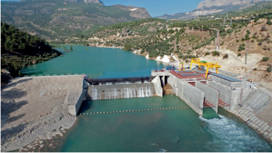
Figure 2. Hydroelectric power plant (ONZATECH, 2014)
