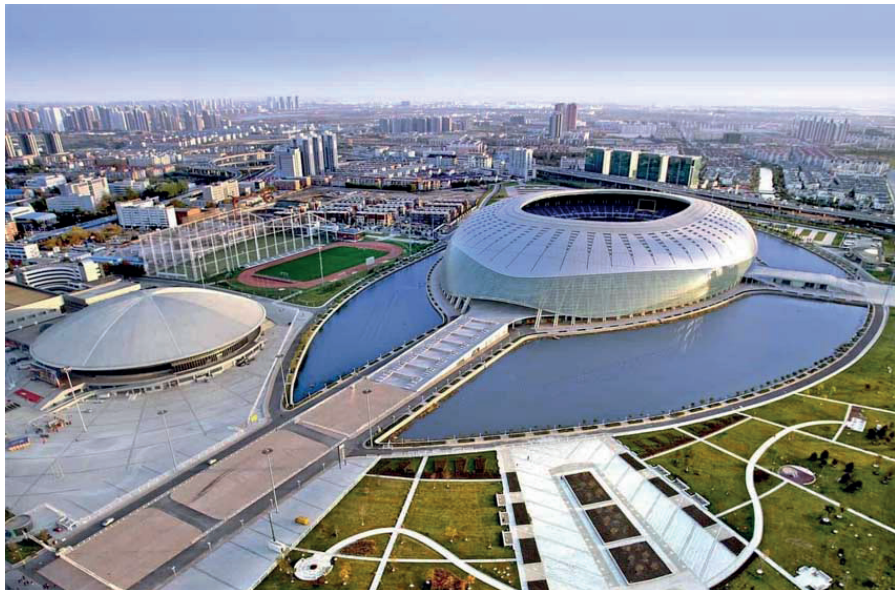
Figure 7. Tianjin Olympic Centre Stadium 19 .
