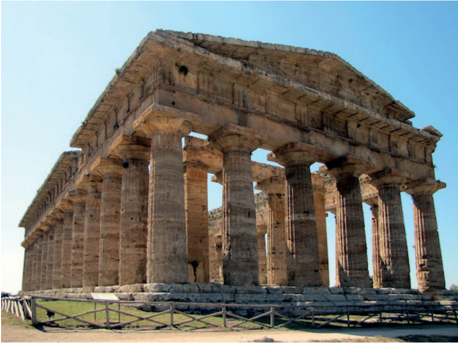
Figure 1. Hera II in Paestum, constructed around 460 B.C.E during the Classical period, is a notable illustration of post and lintel architecture made of tufa and measuring 24.26 x 59.98 meters. 1
