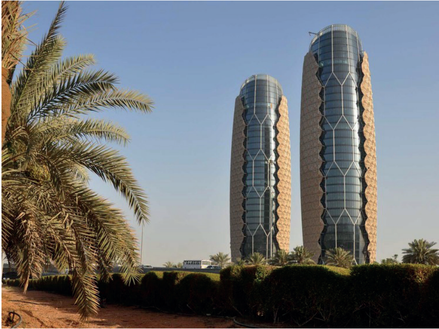
Figure 8. Al Bahar Towers Responsive Facade / Aedas 20 .
