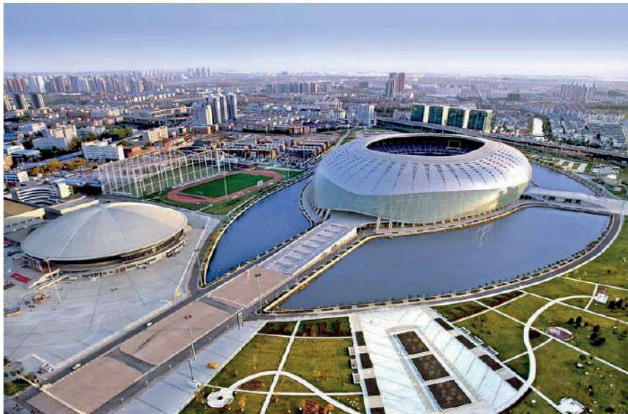
Figure 7. Tianjin Olympic Centre Stadium 19 .
