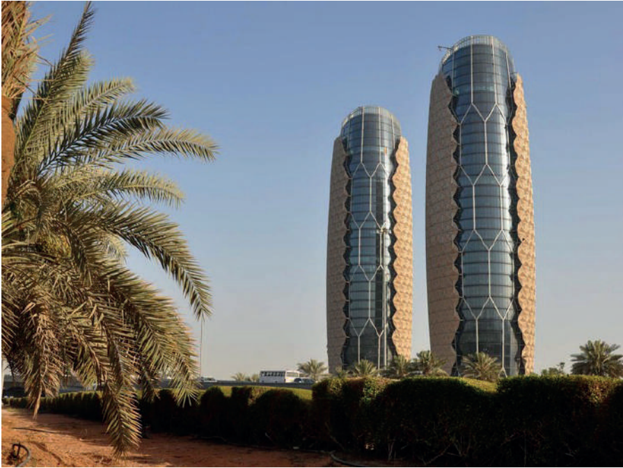
Figure 8. Al Bahar Towers Responsive Facade / Aedas 20 .
