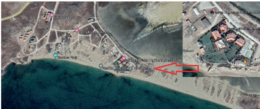
Figure 9. Gökçeada Lagoon, Kefalos beach, Surf Training Centre Application School and other constructions on the beach in the vicinity.
