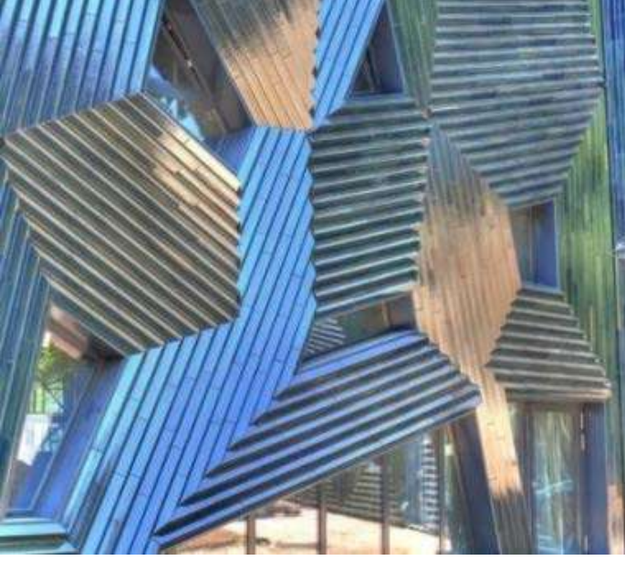
Görsel 22. Manuel Herz Architects of Basel, (Jewish Community Centre Mainz), seramik dış cephe kaplama bina. (İçemer, 2015:34).
